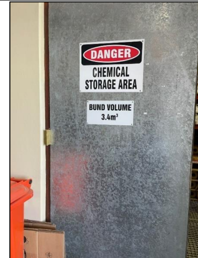
4. Purpose built bunded chemical store
