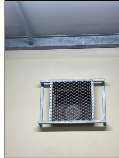
6. Chemical store fitted with appropriate extraction
