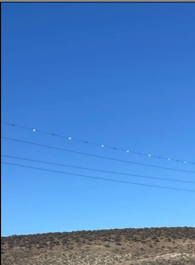
15. Bird diverters fitted to OHL as required
